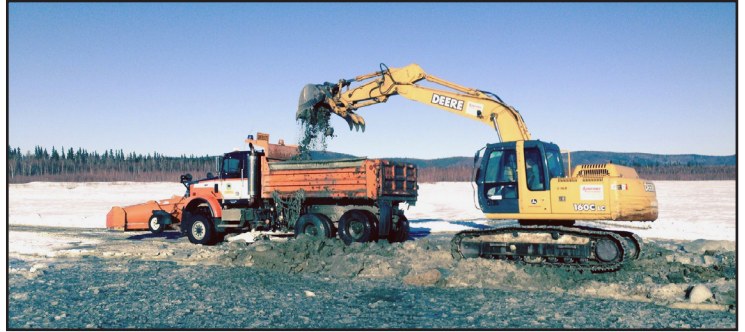
Dredging the boat channel at Harding Lake SRA
